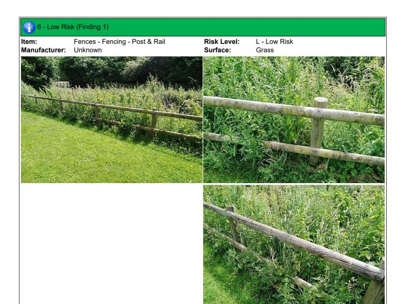
**Finding:** The timber has a number of splits/shakes or air cracks and this may affect the stability or allow water ingress fixing points of the structure and/or cause any instability which will accelerate the rotting process
