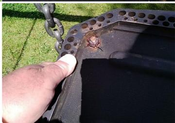
Finding: The cradle seat fixing nuts are corroding
